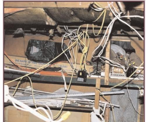
*Modifications to electrical wiring can create a fire hazard.*
